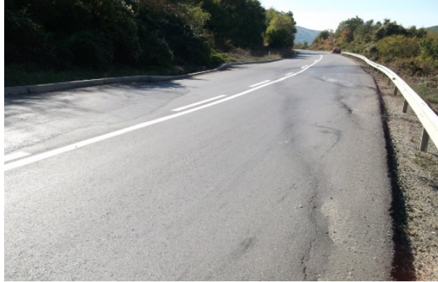
Fig. 2 Skating slot on the regional road Pristina - Gjilan [4]
